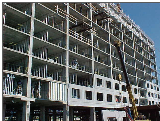
Hyatt Regency Hotel during Precast erection of window boxes.
