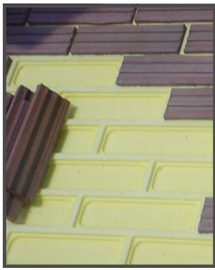
Thin bricks are shown placed in a form liner.
