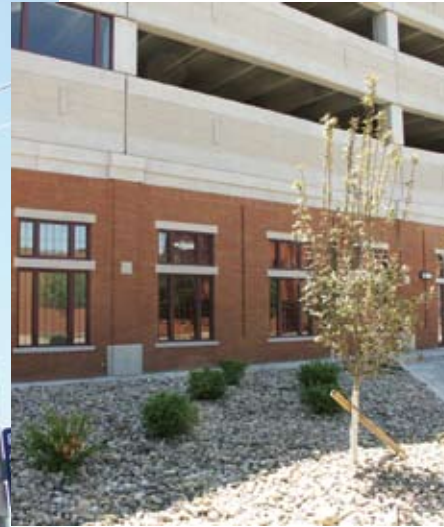
The new Parkersburg, W. Va., intermodal/mixed-use parking facility was produced on a design-build contract. It features an all-precast concrete structural system that helped meet the deadline and budget.
