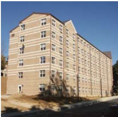
This 400-room dormitory at Fairmont State University was completed in 13 months, thanks to the design-build process. The project features precast concrete hollowcore slabs, which sped construction and saved material.
