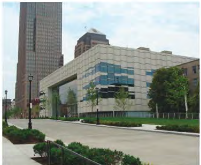
The architectural panels are slightly off-white with a light sand blasted finish on the pixilated profile panel. The precast count on the project was 668 pieces.
