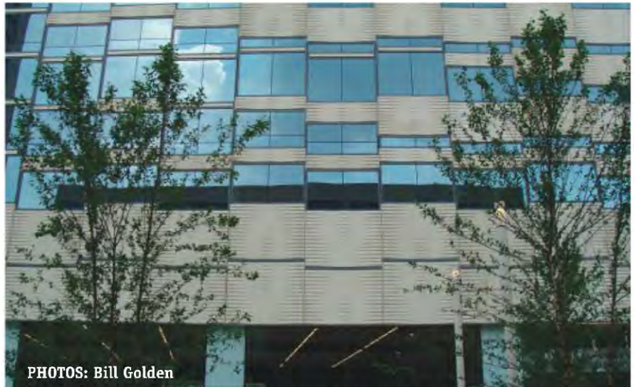
The architectural panels are slightly off-white with a light sand blasted finish on the pixilated profile panel. The precast count on the project was 668 pieces.
